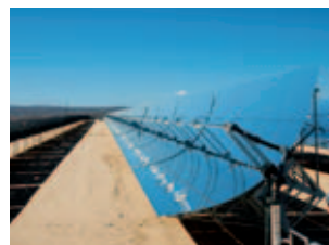
Concentrated solar power applications. Typically large area mirror arrays. Requires a large area and lots of sunshine. Particularly effective in sunny deserts.
