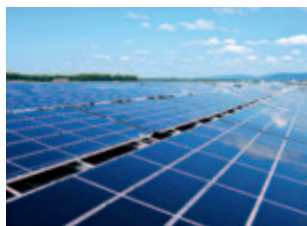
Thin film photovoltaic solar modules produce power at low cost per watt, but require large surface areas for installations.
