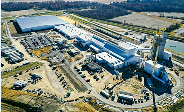
Drone photo of the plant
