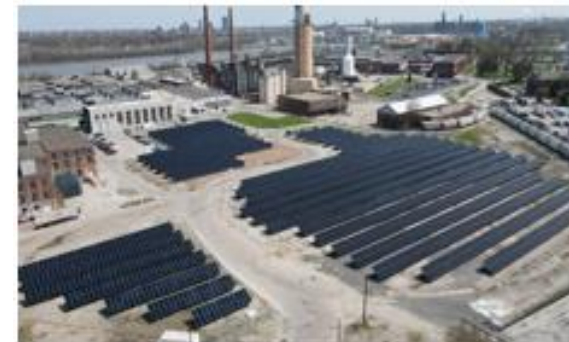
↑ Glass for thin film Solar panels Rossford Solar Array, USA
