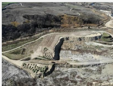
Re-filling and restoration of the sand quarry at Melfi
