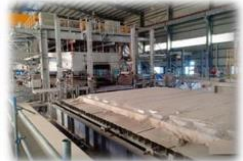
↑ Equipment installation in Vietnam
