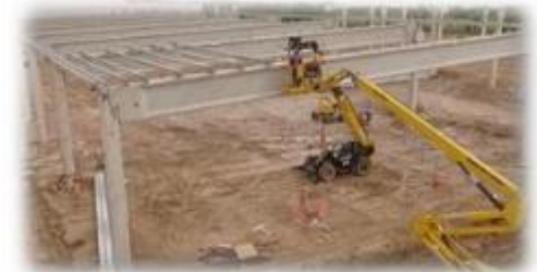
↑ Building construction in Argentina
