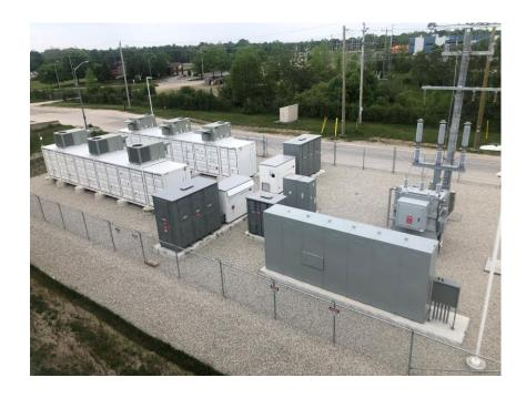
Above: The batteries reduce how much power the Collingwood plant pulls from the grid whenever peak times are predicted.
