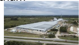
New float furnace in Argentina
