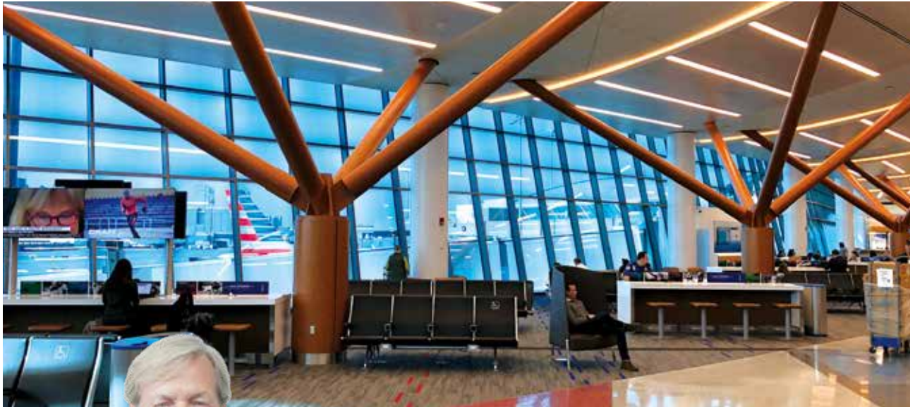
The Boston Logan Airport installation, Electrochromic windows by View, Inc. with NSG Group TEC™ glass
